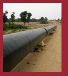
The Mangala Development Pipeline in India requires a constant, elevated temperature above 149°F (65°C) to ensure flow of crude oil over a distance of 400 miles (700 km). Pentair's Thermal Management business engineered and bundled multiple state-of-the-art technologies, delivering a one-of-a-kind, safe, reliable, cost-effective, and energy-efficient system, helping create the world's longest continuously heated and insulated pipeline.
